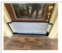
Front Door Sealed same process as garage door. But we also strapped this front door with strap see picture below to stop door from being pushed in by water.
