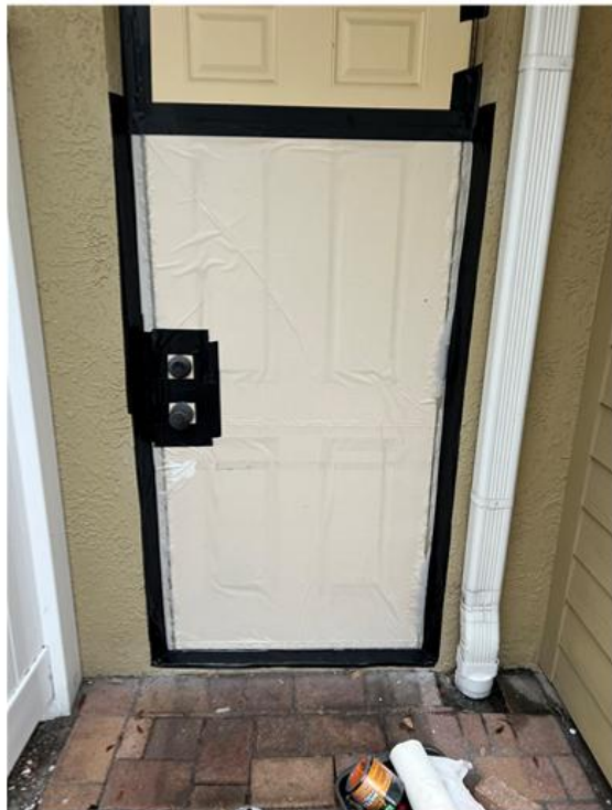
Main Garage door sealed with seal n peel, 3M spray on all edges to hold 6 mil plastic sheeting, gorilla tape all edges. Reason for different color tapes is we ran out of gorilla tape, normally would use all gorilla tape.
